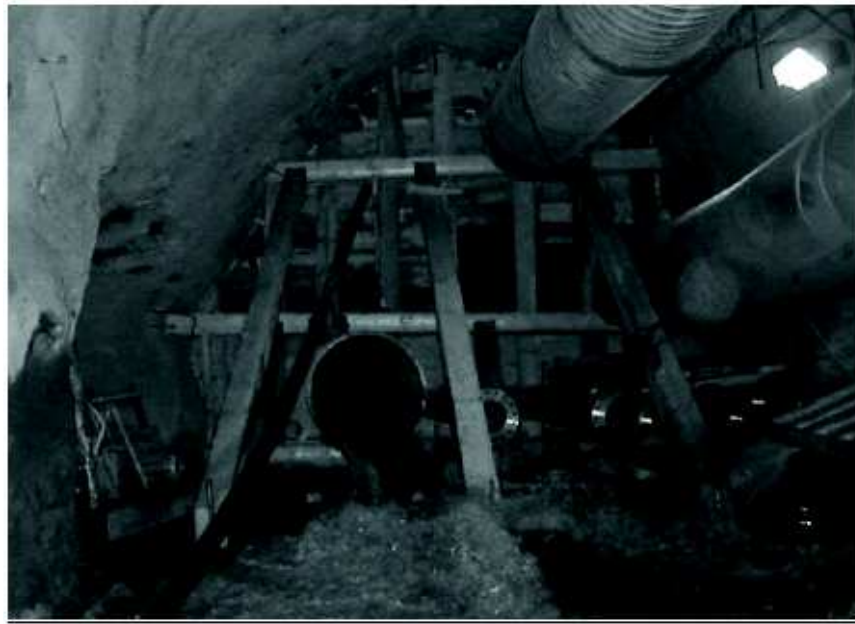
Figure 7- Initial timber bulkhead wall
