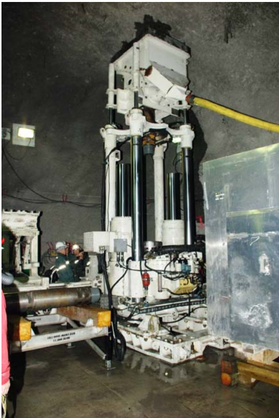
Figure 5 Boxhole drill, and drill chamber set up (McArthur River Operation, 2010)
