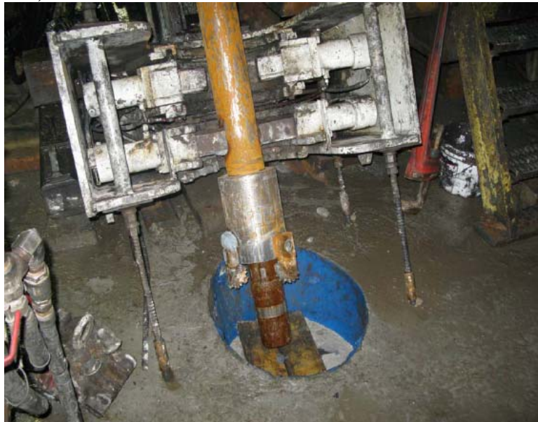
Figure 7 Overcoring bit and set up for freeze hole removal (Cameco Clarifier, 2009)
