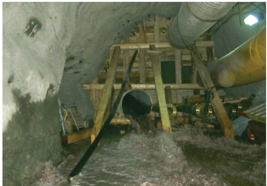
Figure 6. Initial timber bulkhead wall, McArthur River.
